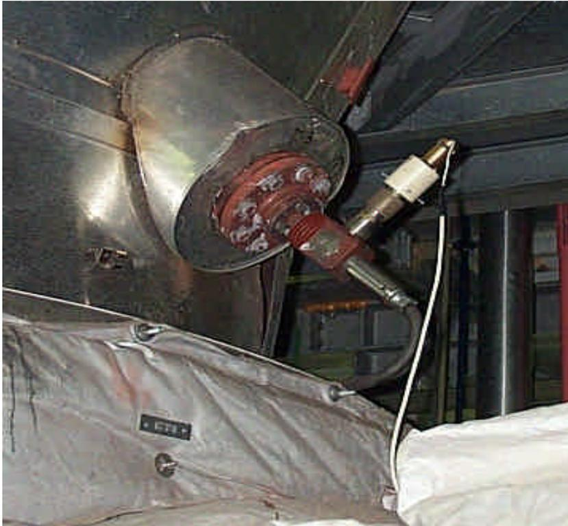
**Figure 5.** Installation of optical sensor.
